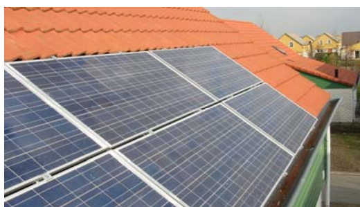
Figure: PV modules installed between the tiles (left) and above the tiles (right)
